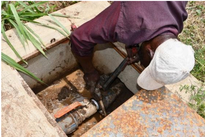
a civil engineering student fixing a manhole valve leakage
